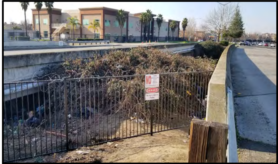
Figure 1 – Truxel Road Bridge
