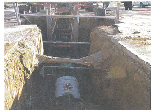
Replacing 50-year-old storm drain infrastructure ▲
