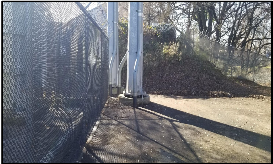
Figure 4 - SMUD Substation Encampment
