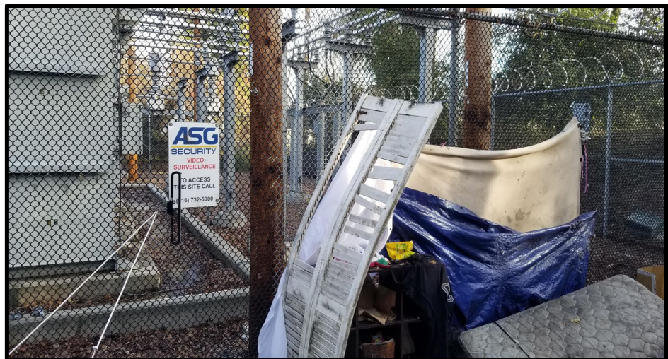
Figure 2 - SMUD Substation Encampment
