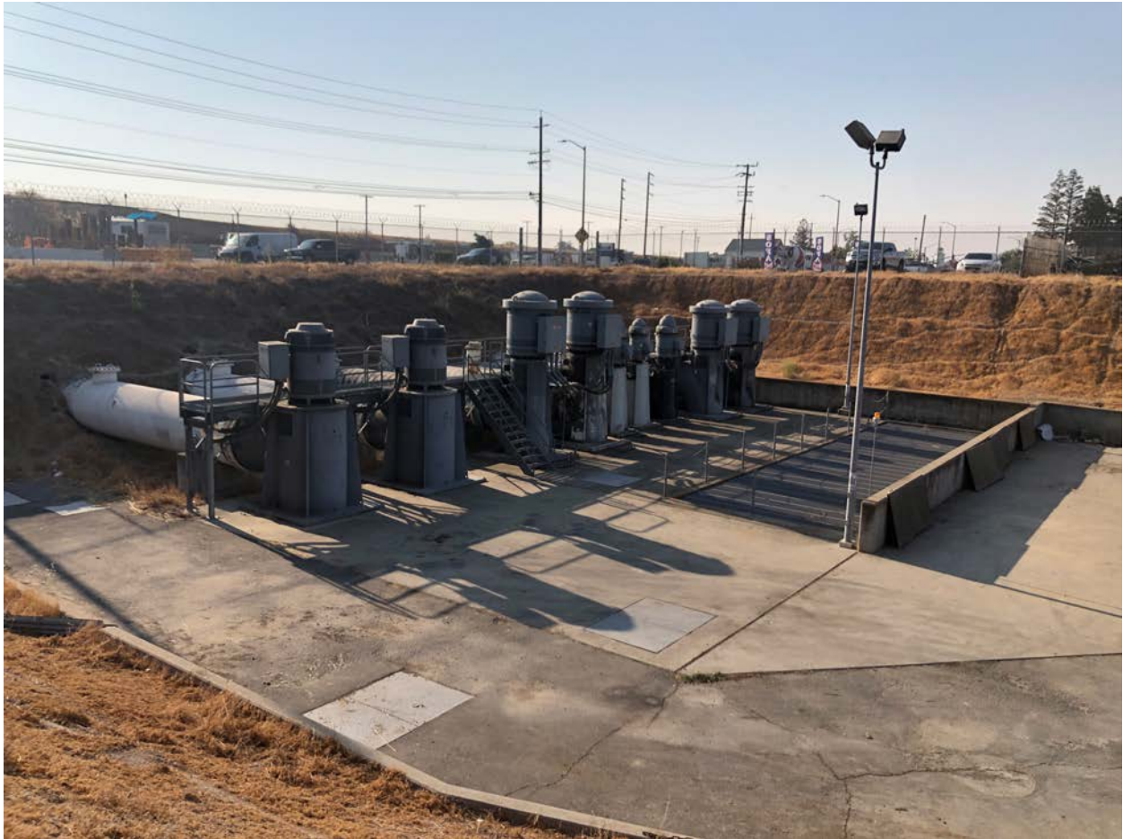
Figure 1. Photograph of the RD1000 pump station
