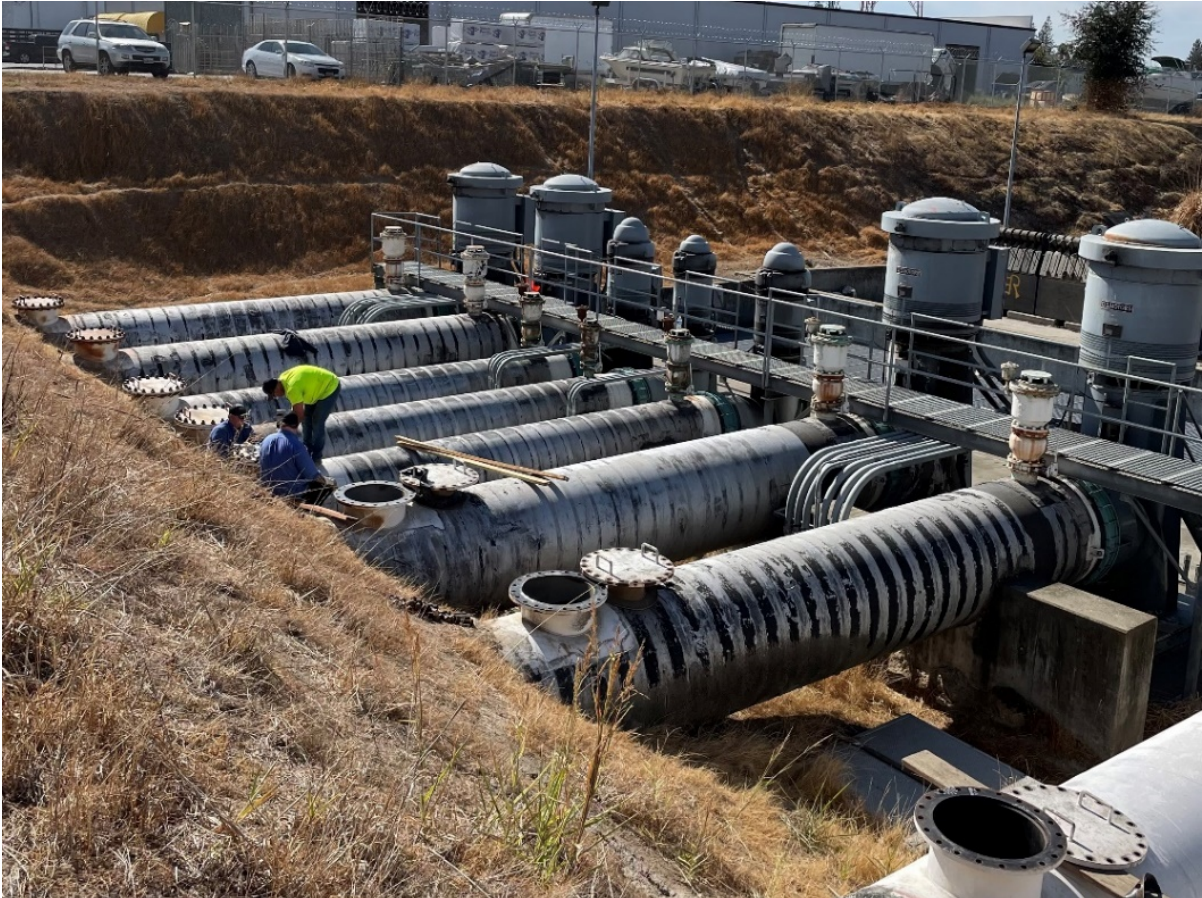
Figure 4-1 CCTV Pipeline Inspection
