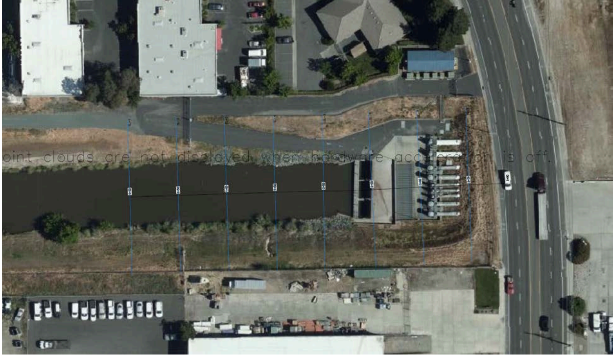
Figure 2. Photograph of the RD1000 pump station (plan view)
