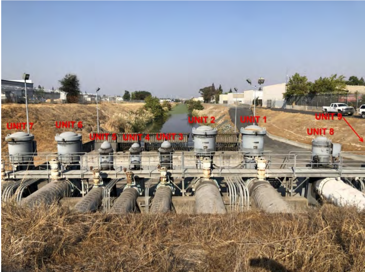
Figure 1 RD 1000 Pumping Plant 8 Looking West Towards the Drainage Canal
