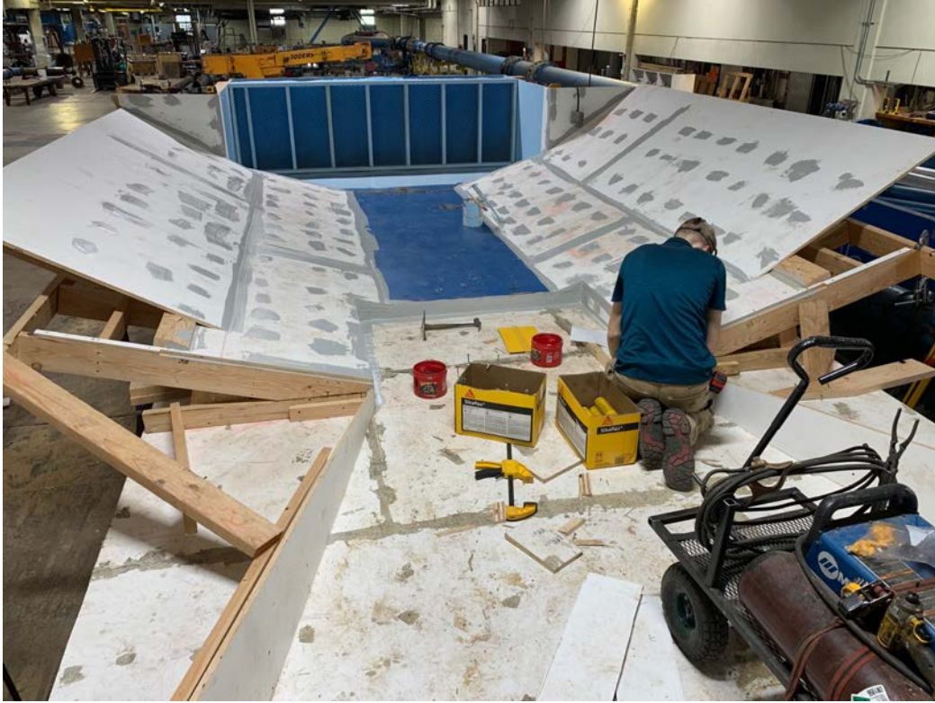
Figure 7. Physical model during construction
