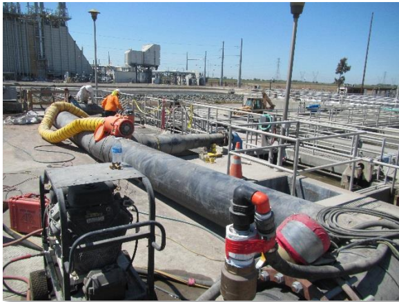
Photo 2-1. Example of HDPE bypass piping system installed.
