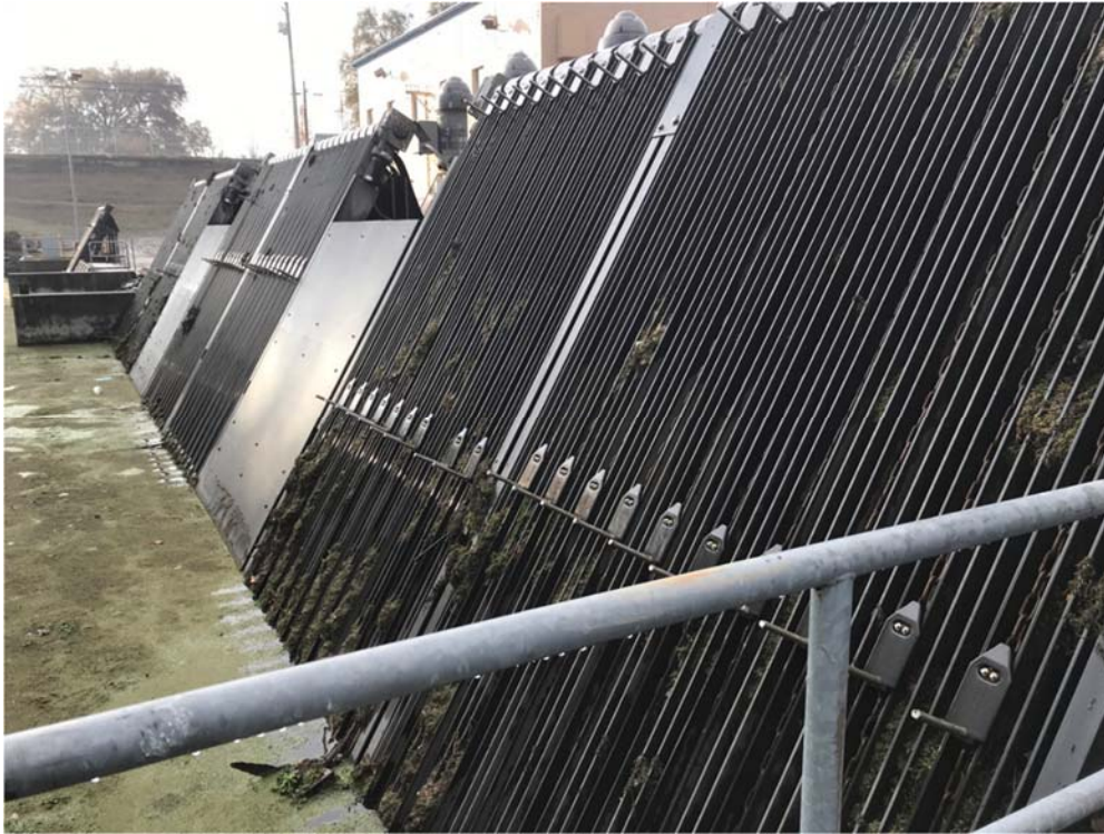
Figure 3 - Pumping Plant 1B Intake Screens
