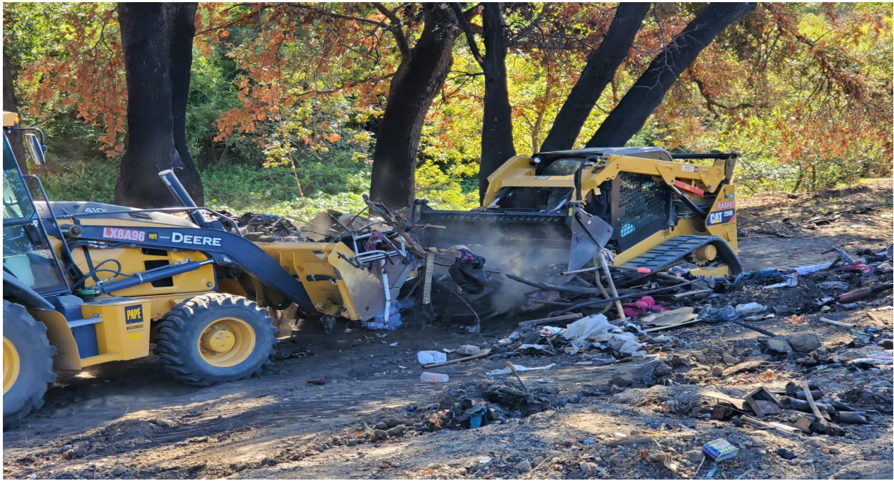
A bakchoe and skid steer working together to gather trash.
