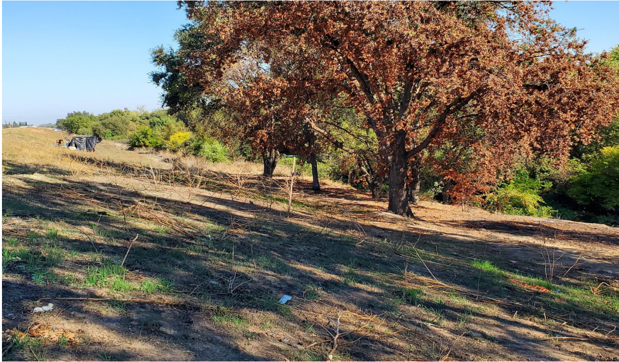
A picture of the newly restored levee slope and toe.
